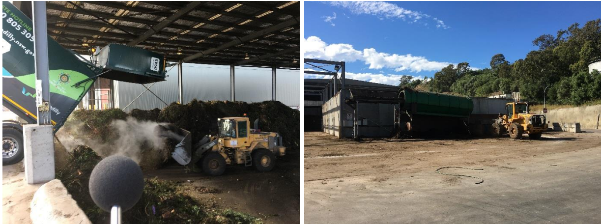
Figure 3: Organics Reception (left) and Tunnel & Trommel (right)
