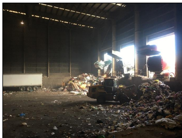
Figure 2: Inside ARRf Waste Bulking
