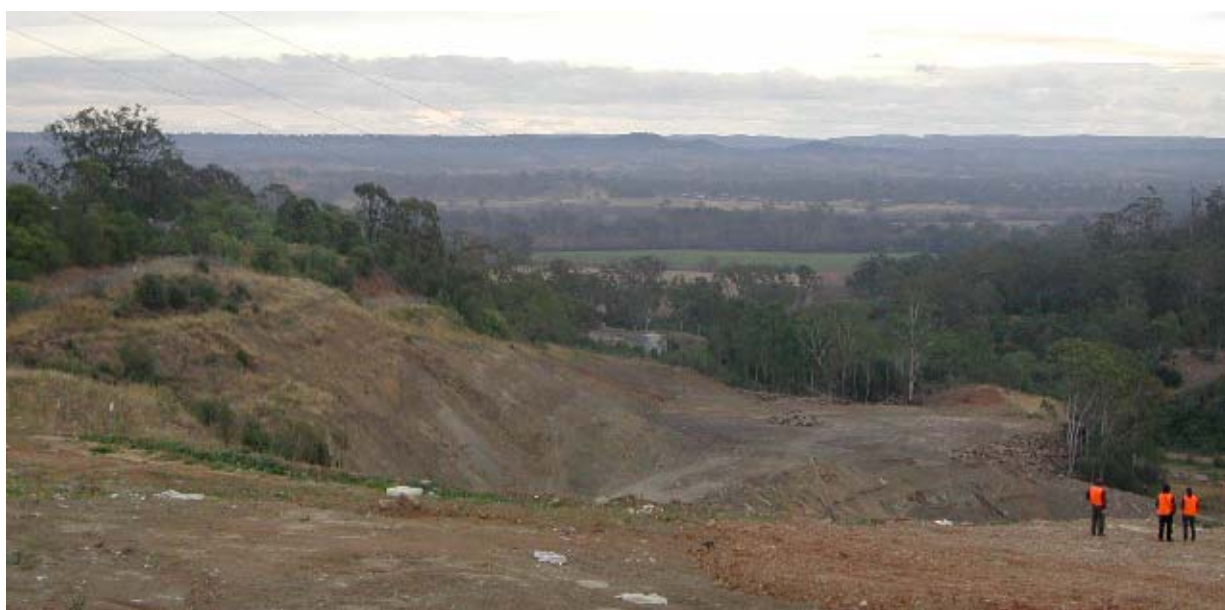
Figure 8 Embankment on east and south of site for proposed development.
