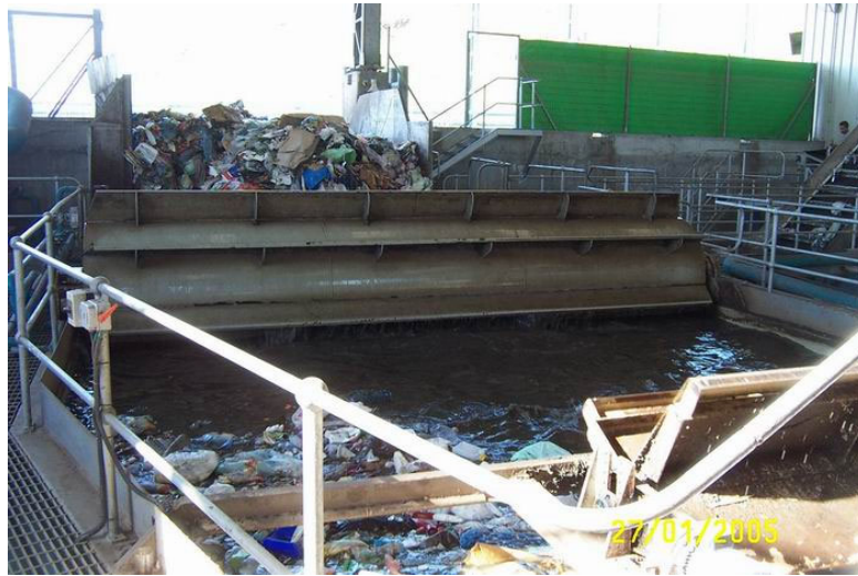
Figure 5-6 Vat and waste dropoff area
