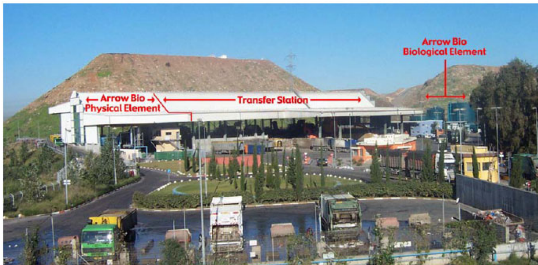
Figure 5-1 ArrowBio plant in Tel Aviv, Israel
