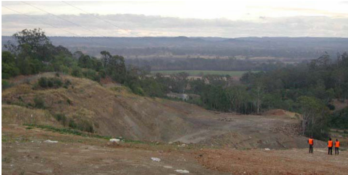
Figure 16-4 Embankment on east and south of site of proposed development.
