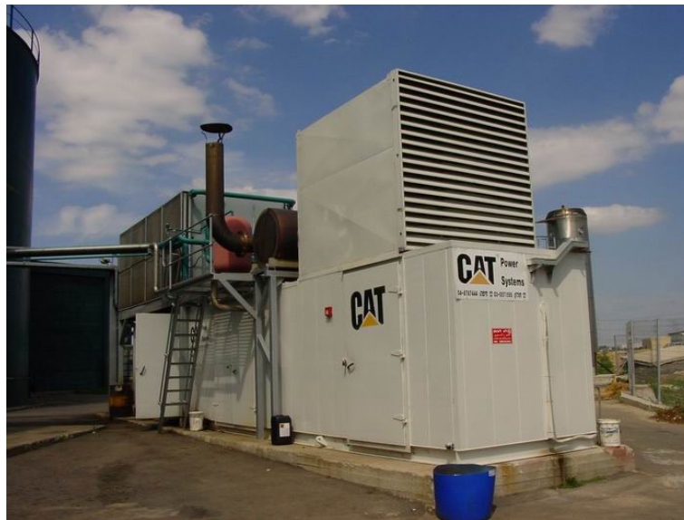
Figure 5-10 Gas engines
