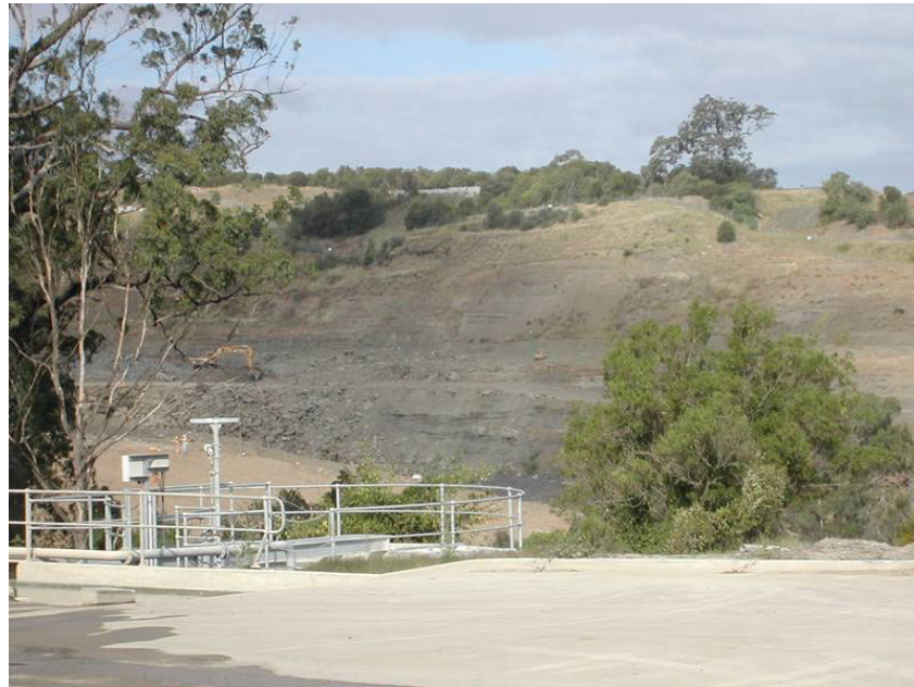
Figure 1-4 Location of proposed AWT Facility as viewed from existing operational area
