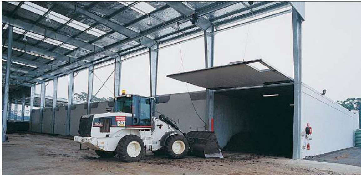
Figure 5-20 Unloading of compost from tunnels at the Port Macquarie facility
