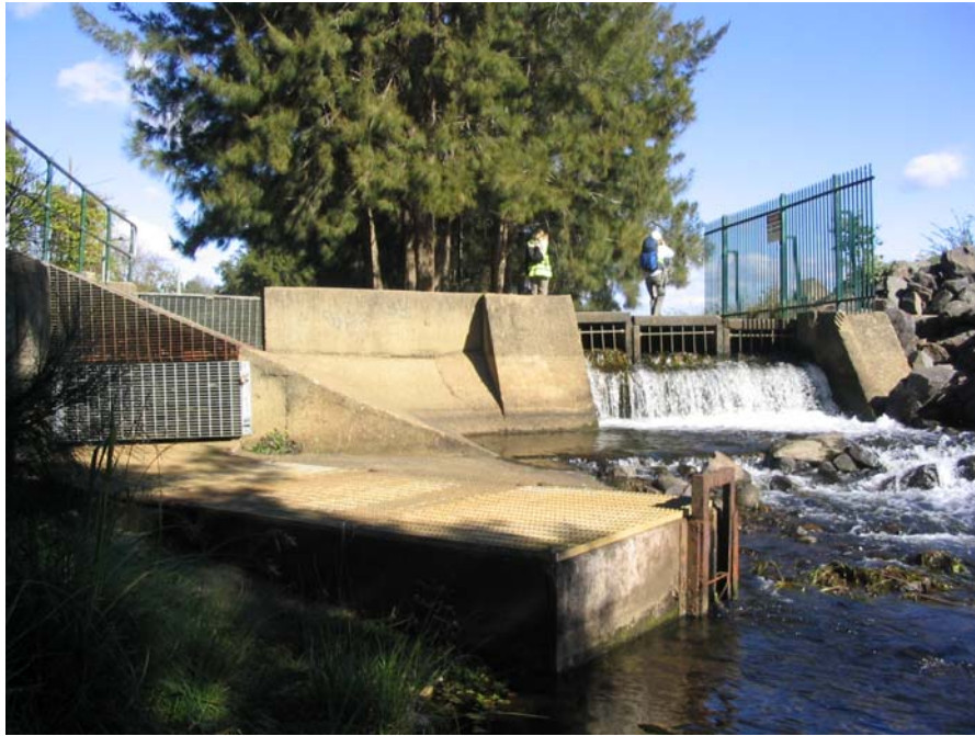
Plate 1: Fish ladder (foreground) and overflow of the Penrith Weir
