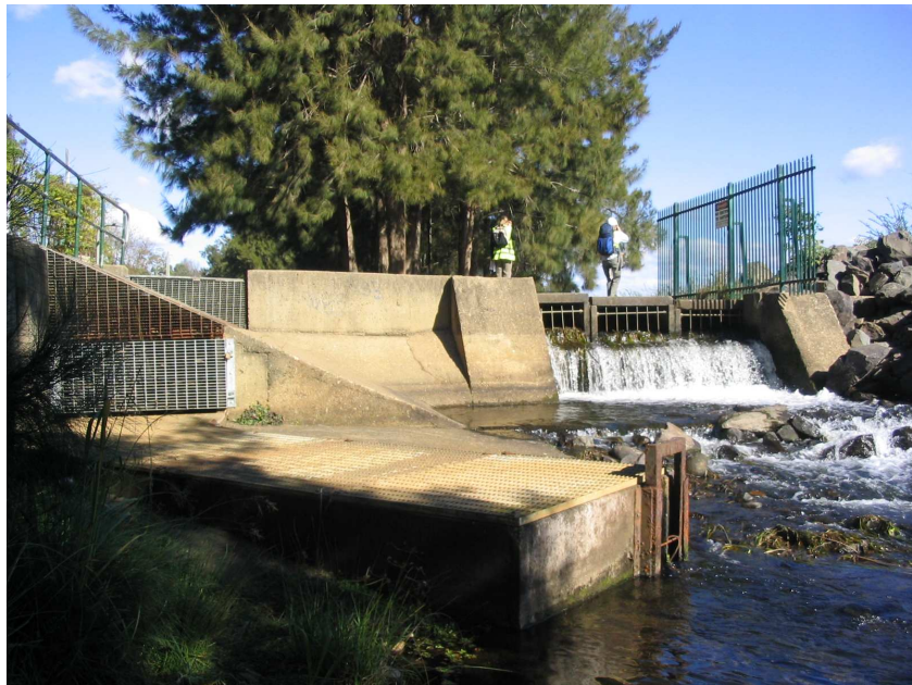
Plate 2: Fish ladder (foreground) and overflow of the Penrith Weir
