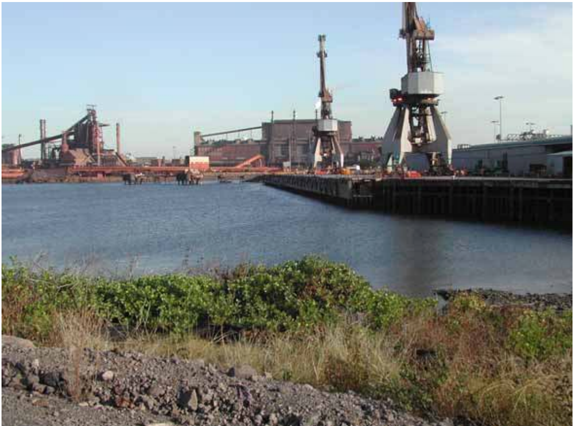
Plate 3-1: Looking south towards the Existing No. 2 Products Berth and BlueScope Steel
