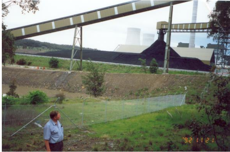
Plate 5 – Mt. Piper Power Station Coal Stockpile
