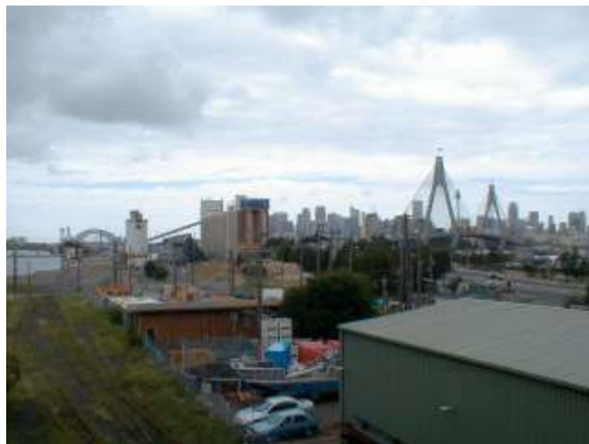
↑ Northern view of Silos from northern footpath along Victoria Road
