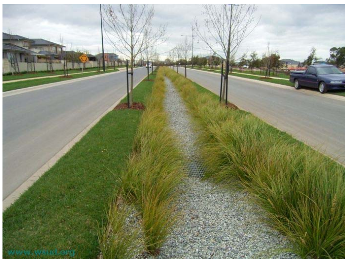
Figure 3.3: Typical biofiltration trench
