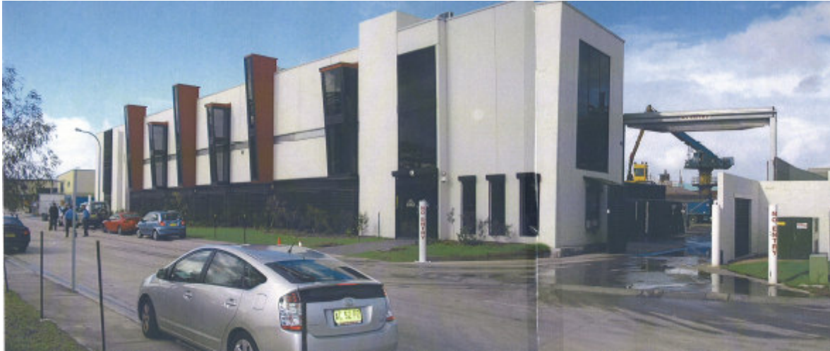
Figure 6: The Sell and Parker facility on Baker Street
