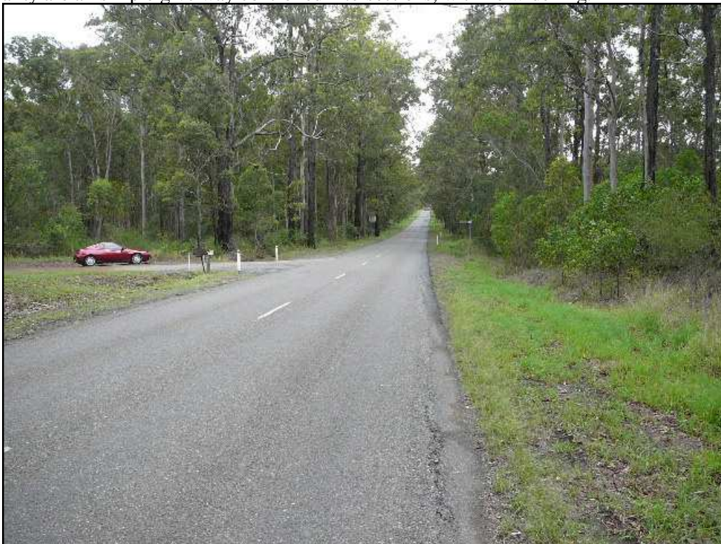
Photo 1 - View east along Bucketts Way showing typical cross section. Note Urray Road is to left of photo.
