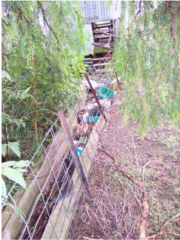
Photograph C: Disused sheep dip at Pine Park.
