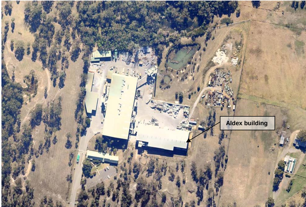
Figure 2: Aerial view of Weston Aluminium's Kurri Kurri Facility
