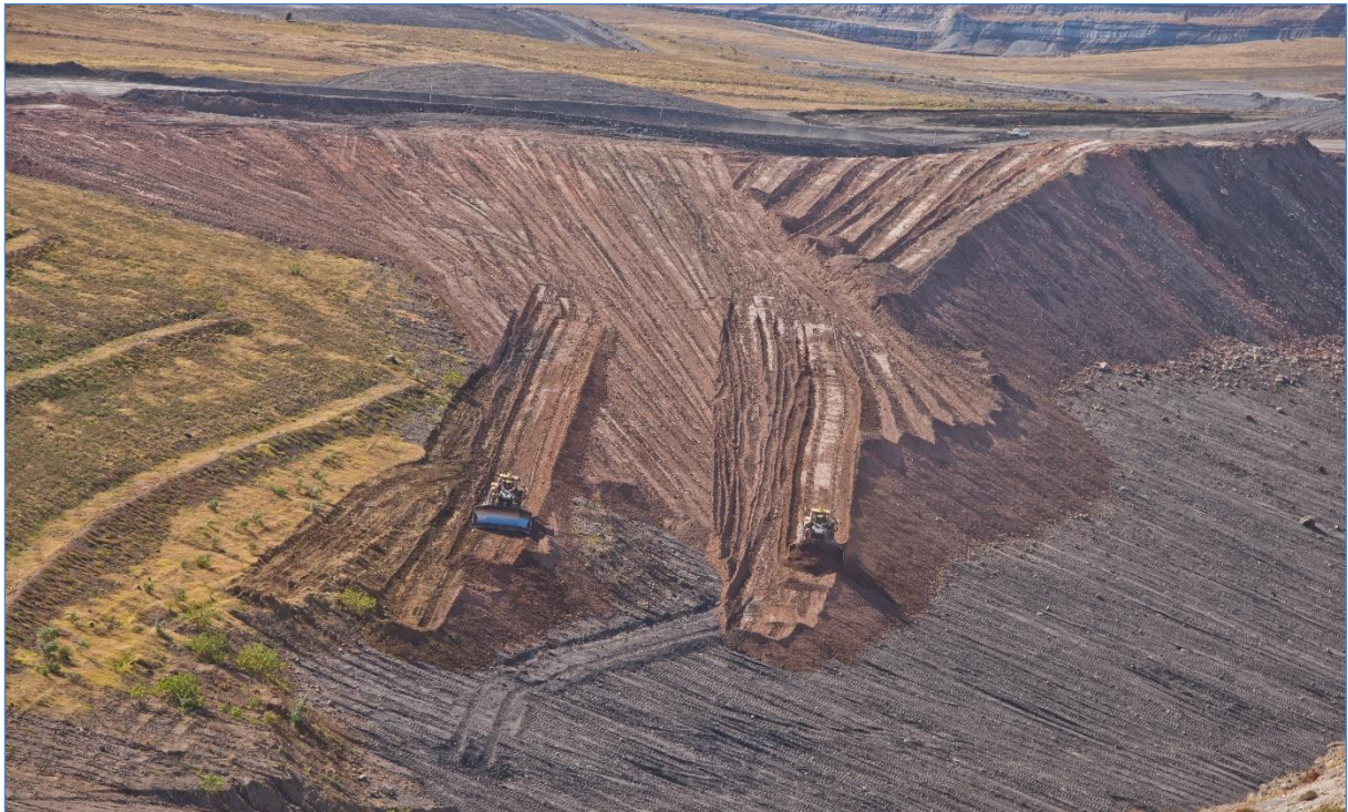
Plate 4 – Malabar’s Rehabilitation Activities in CL 229 (Spreading of Inert Capping Material)
