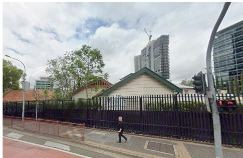
North west view to Lancer Barracks from Station Street East showing boundary fencing
