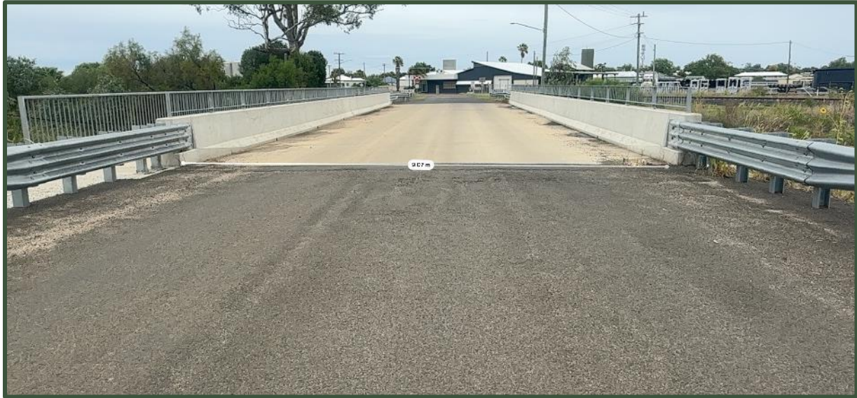
Figure 9 Nearby Bridge (Horsearm Creek)
