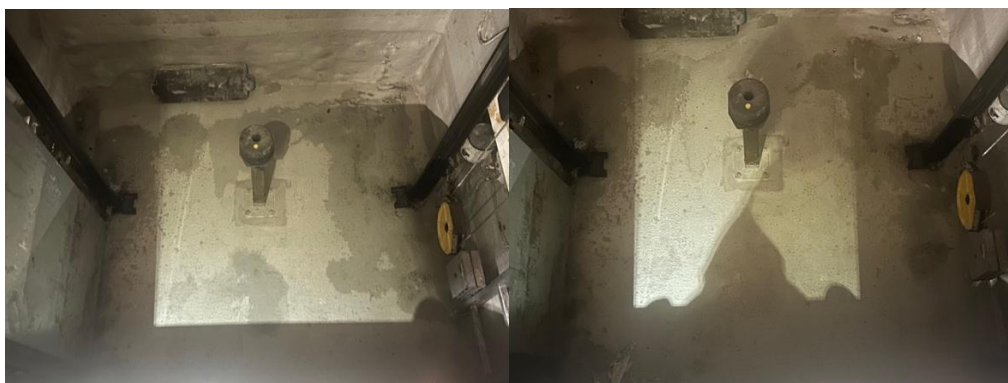
Left and below: Lift shaft flooding and basement water ingress – Wilberforce Ave (2025). Photos supplied by residents
