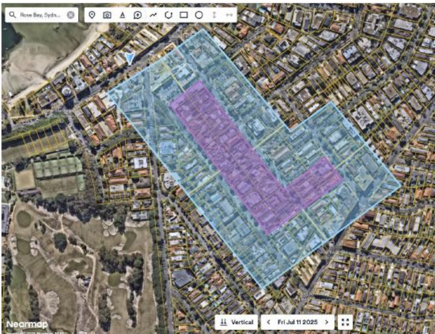
Plate 4-4: Aerial Photo Showing the Approximate Area That will be Impacted by Groundwater Drawdown During Dewatering if All Proposed Developments Were to Proceed
