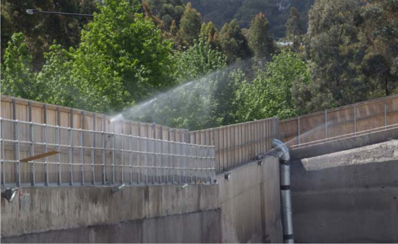
Figure 11 - Dust Mitigation at Norwest Station Site
