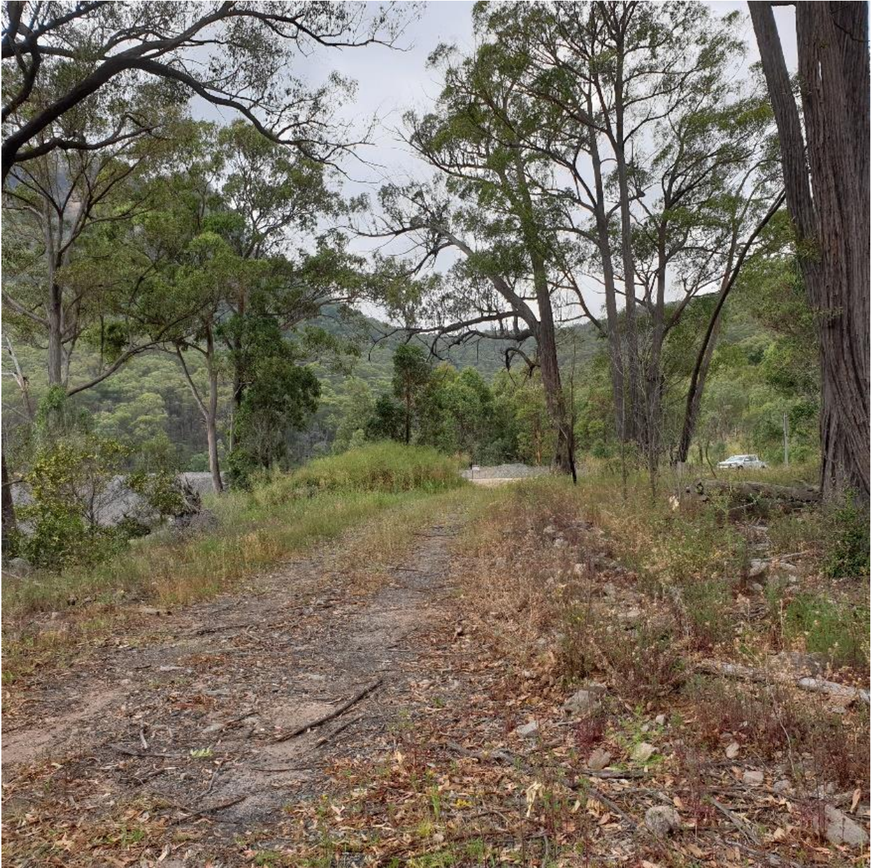
Plate 1 Area of road to be widened in PCT 1088
