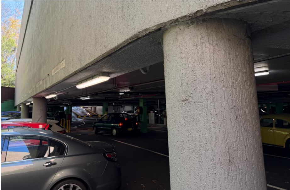
Figure 6 – Coles Underground Carpark Lighting
