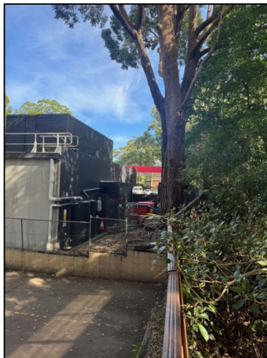
Figure 43: Tree 32 – Note the excavation in TPZ in adjoining site.
