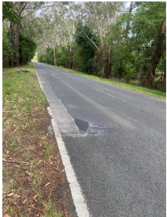
**The worst section of road – photos taken at different angles to try and show the height of the “shoving” in the middle of the road – this section is dangerous and would be especially so to smaller vehicles**
