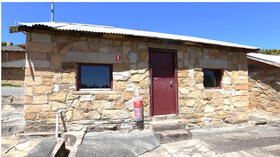
Figure 13 Sandstone and brick garden sheds located outside the Gaol wall on the south.
