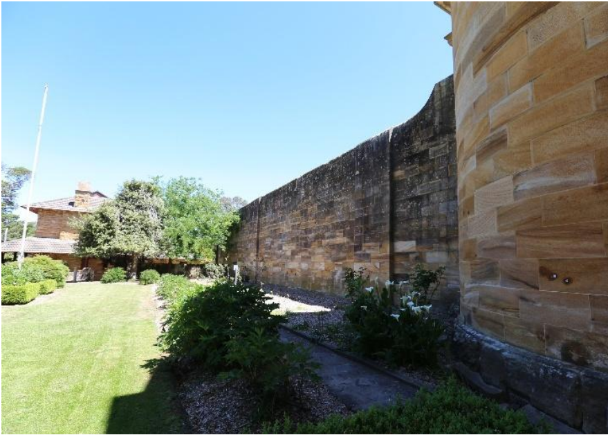
Figure 9 View alongside the eastern wall of the Gaol.
