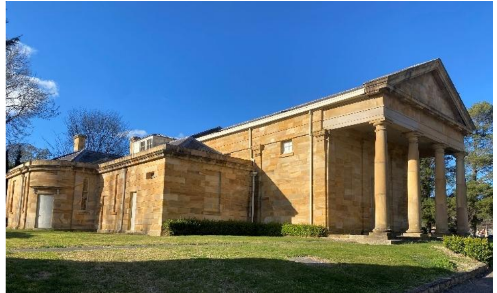
Figure 6 Berrima Court House, located at the junction of Wilshire Street and Argyle Street.
