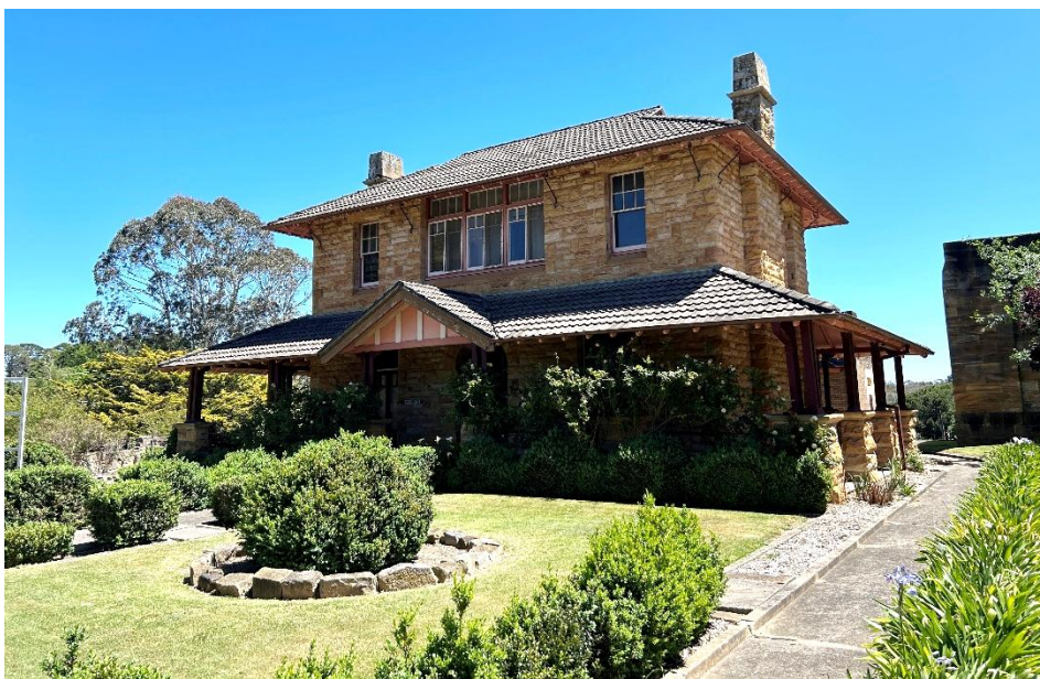
Figure 14 Former Governor's residence and front garden, facing Argyle Street.
