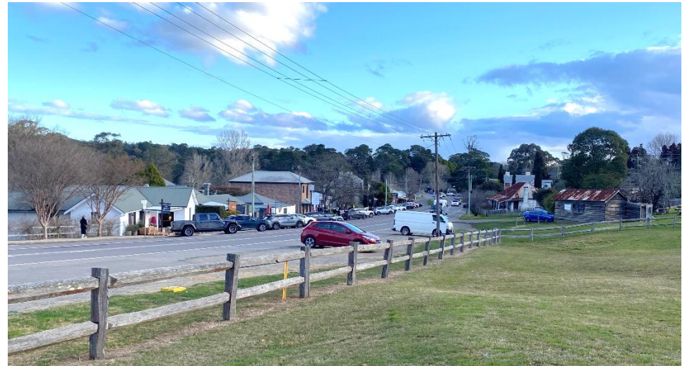
Figure 7 View south into the town centre of Berrima, at corner of Old Hume Highway and Oxley Street.
