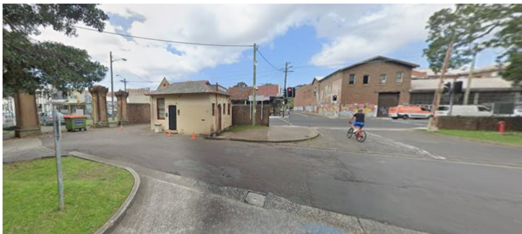
Figure 3.17 Existing structures (Balmain Road park entrance)
