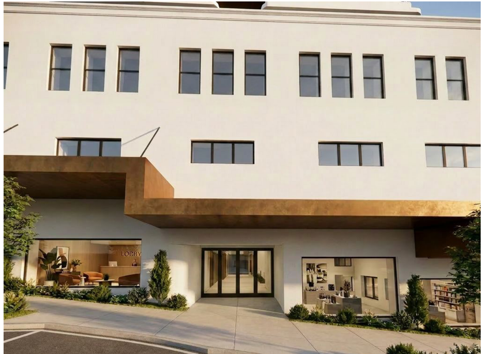
BUILDING 01 ATCHISON STREET ENTRY
