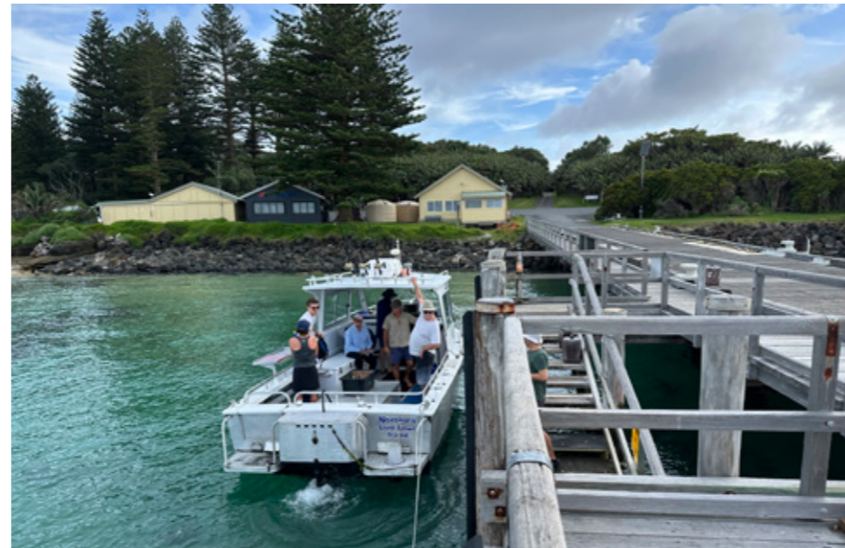
LC2 - Marine Infrastructure
