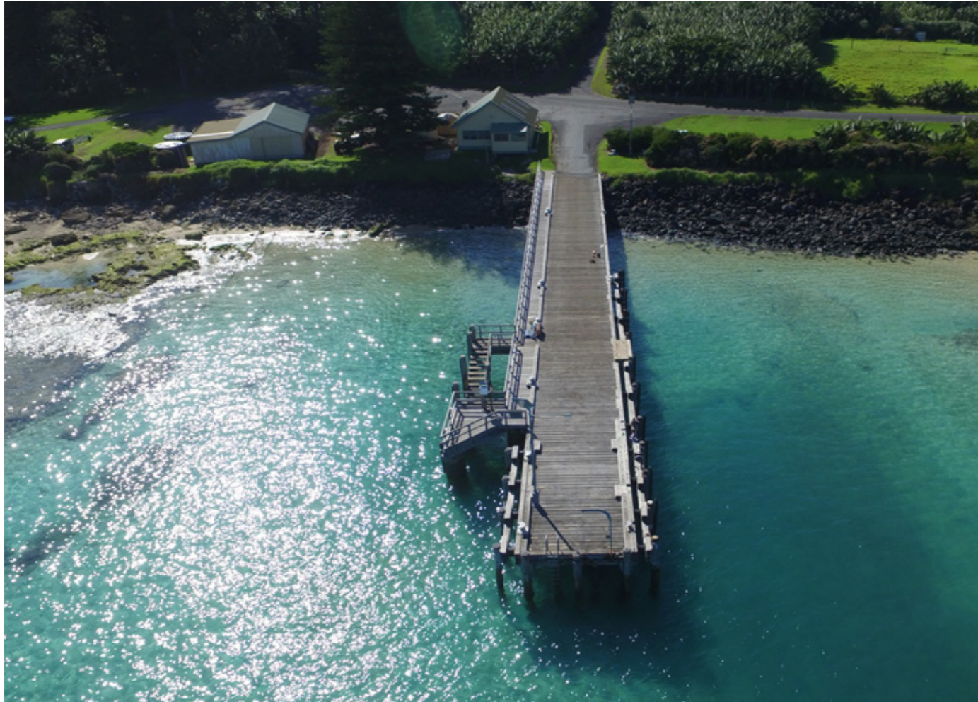
Figure 19: NZ Drone Imagery of the jetty and adjoining buildings
