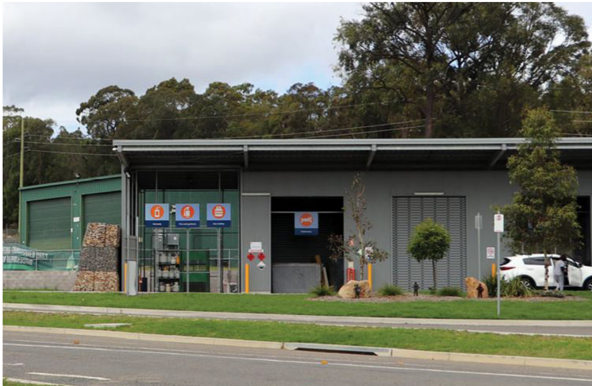
COMMUNITY DROP OFF SHED
