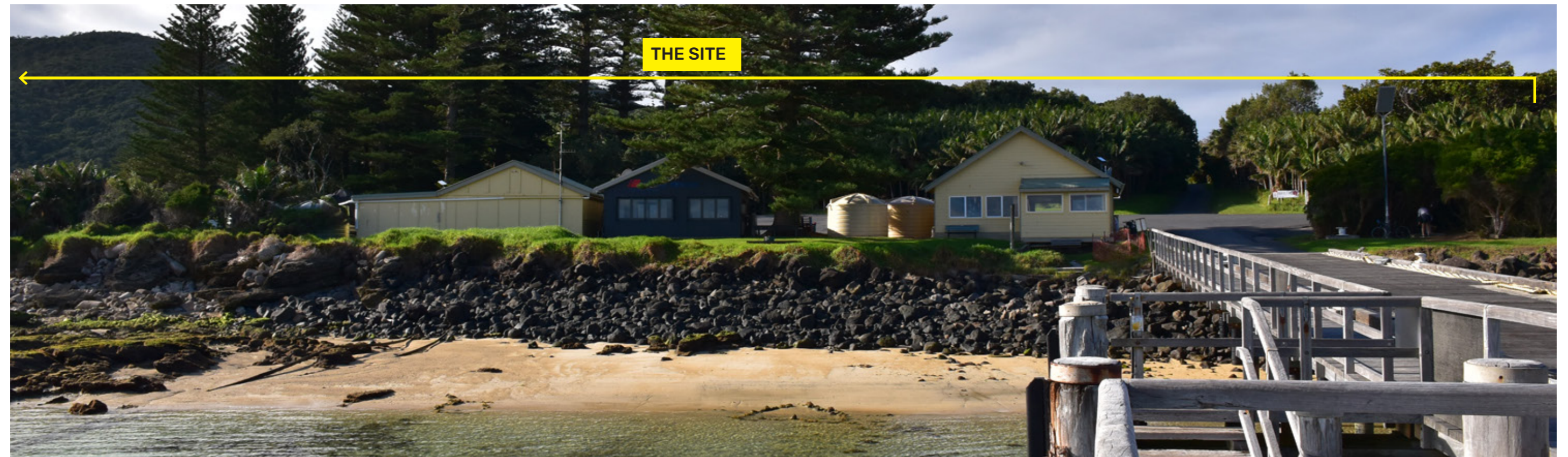
Figure 88: Viewpoint 3B - Existing Jetty
