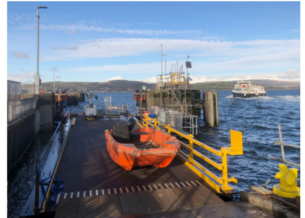
Figure 48: Example of a Linkspan (RoRo)
