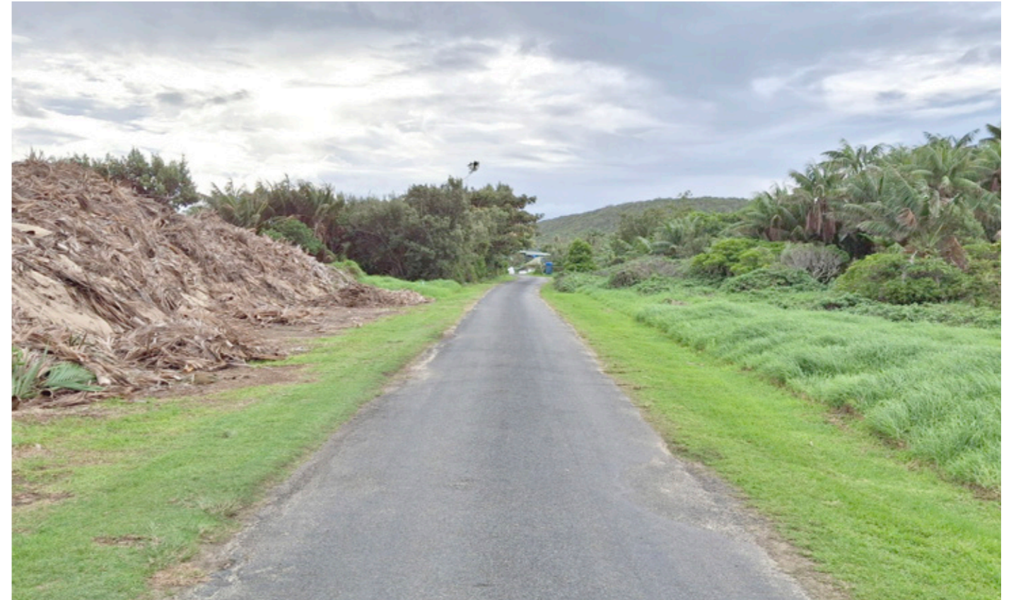
Figure 34: Public driveway into Waste Management Facility
