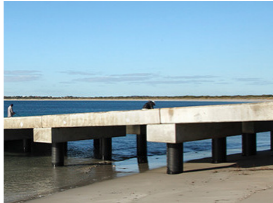
Figure 47: Example of a Fixed Piled Ramp (RoRo)
