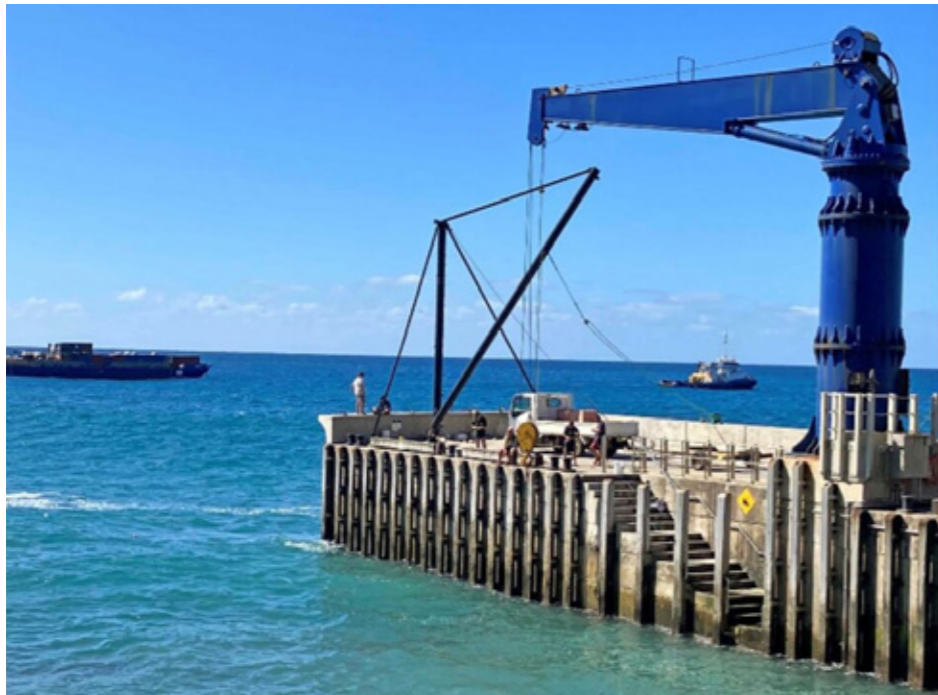
Figure 46: Example of a Pedestal Crane and Jetty (LoLo)
