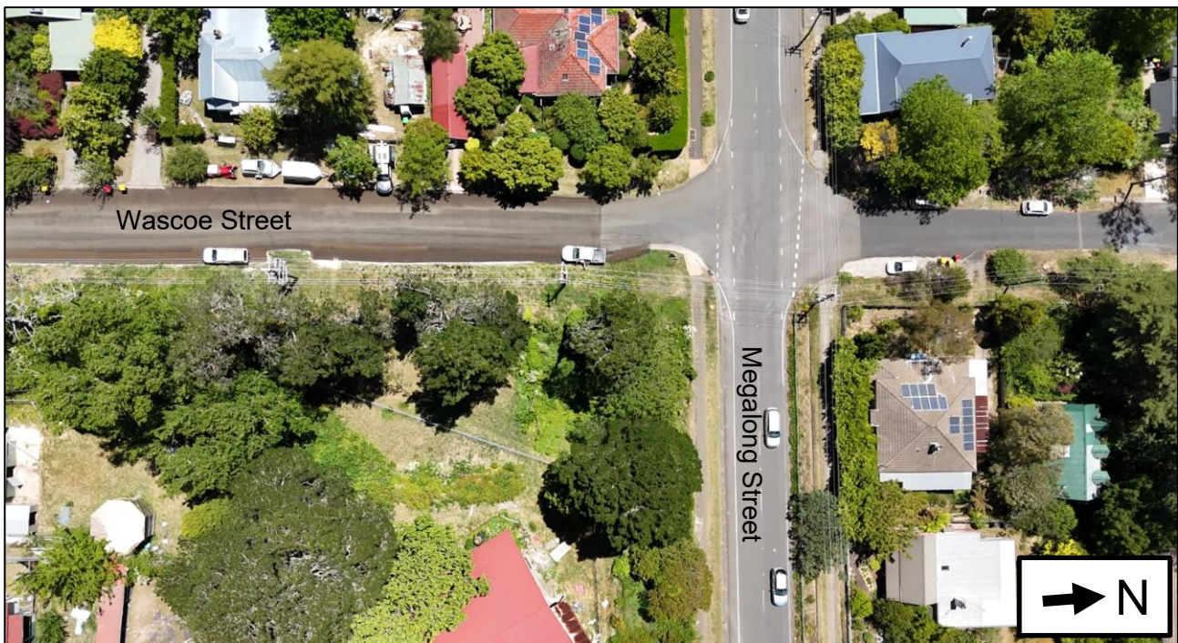
FIGURE 1: AERIAL IMAGE OF WASCOE STREET RECENT ROADWORKS
