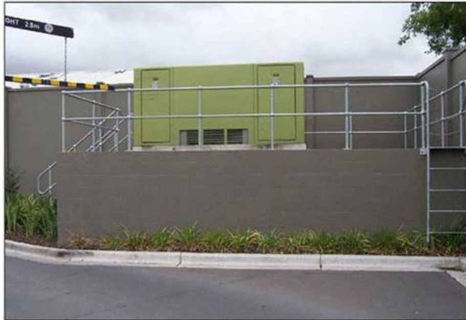
Figure 51 - Example substation raised above 1:100 flood level
