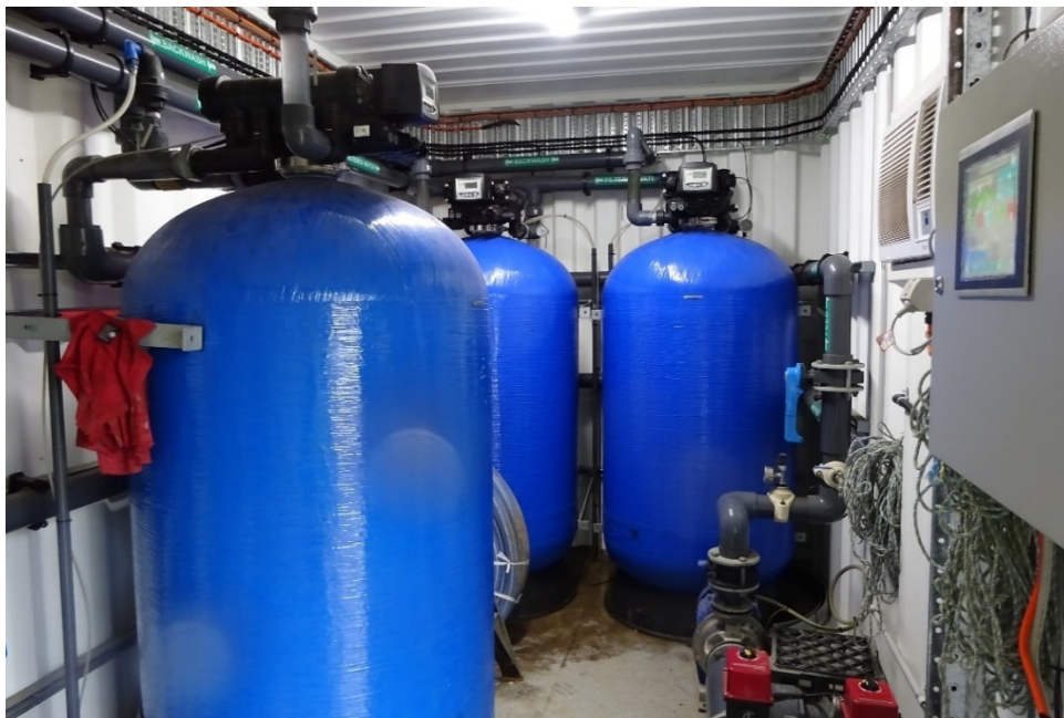
Figure 6 Proposal site's Tertiary Water Treatment System (TWTS)
