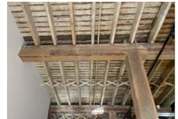
Timber posts from ground floor 'Building 1' per Heritage Assessment Report
