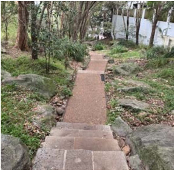
Orphan School Creek Gully Restoration path commencing from Bridge Road
