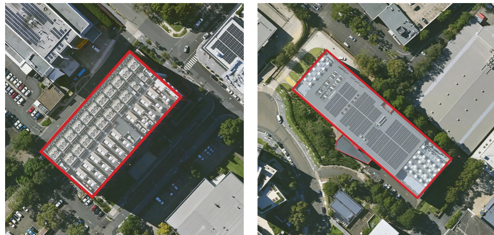
Data centres in Macquarie Park: (Left) 4 Eden Park Drive; (Right) 6/8 Giffnock Avenue
