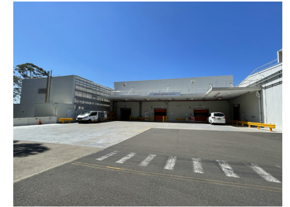
2. Existing warehouse upper level
