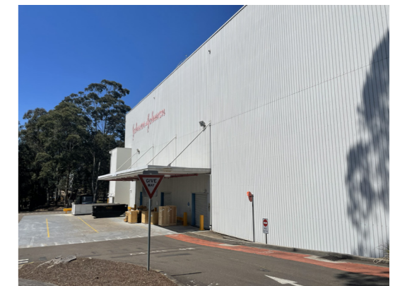
6. Existing warehouse lower level
