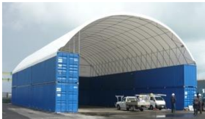
Plate 3.1 Indicative Mobile Processing Plant Enclosure
