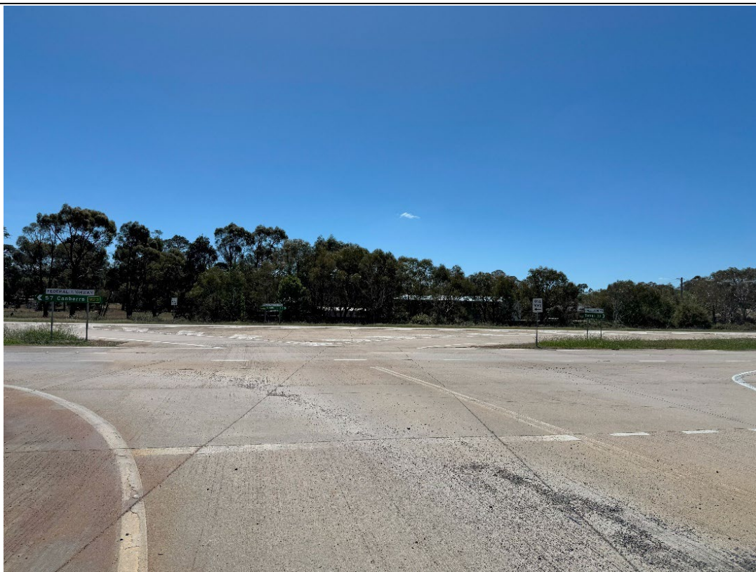
Figure 3 Site Access Federal Highway looking North
