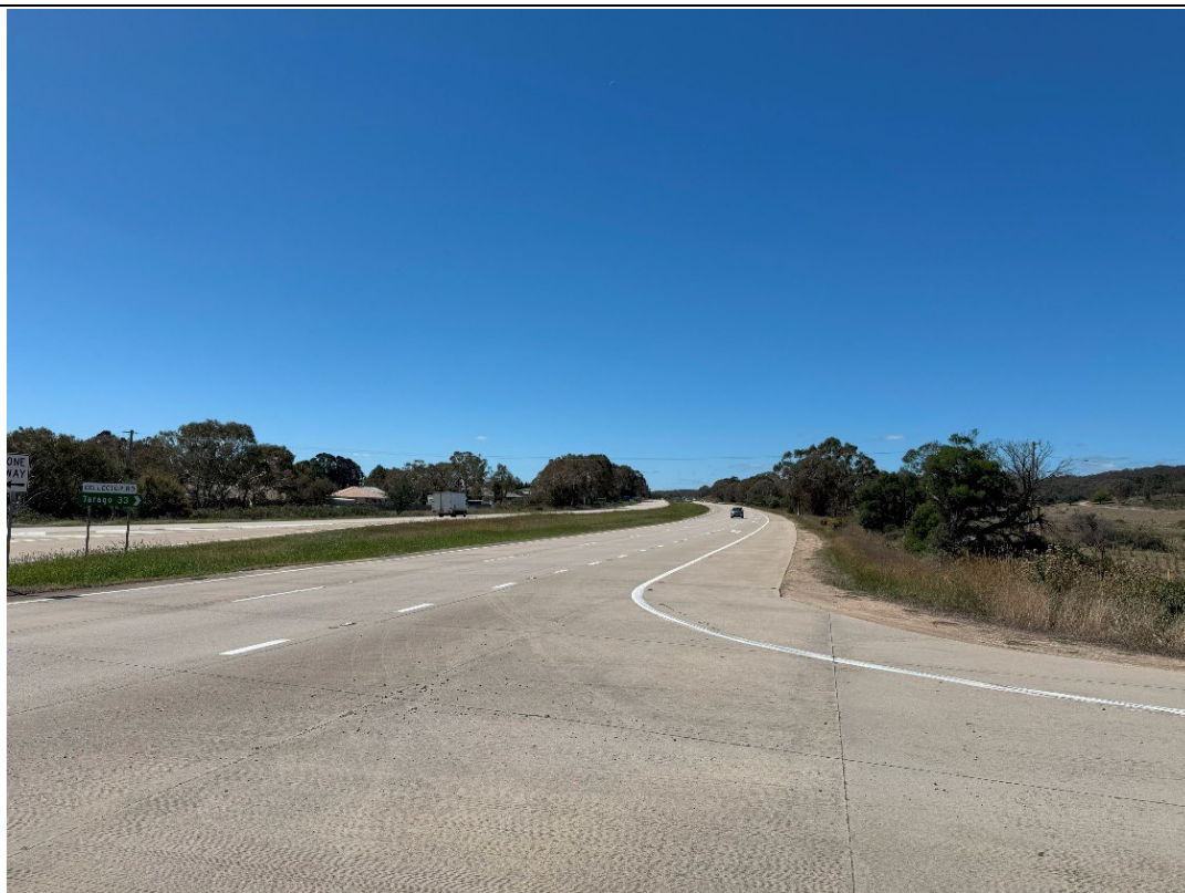
Figure 5 Site Access Federal Highway looking North
