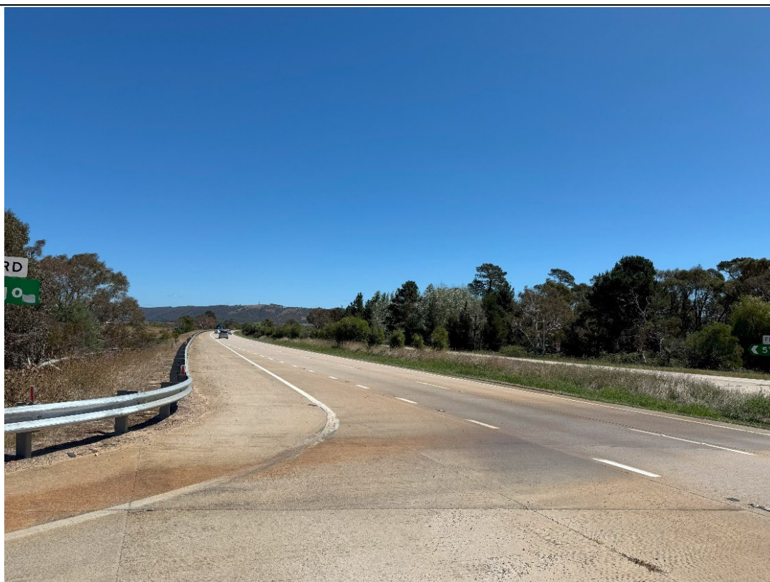
Figure 4 Site Access Federal Highway looking North
