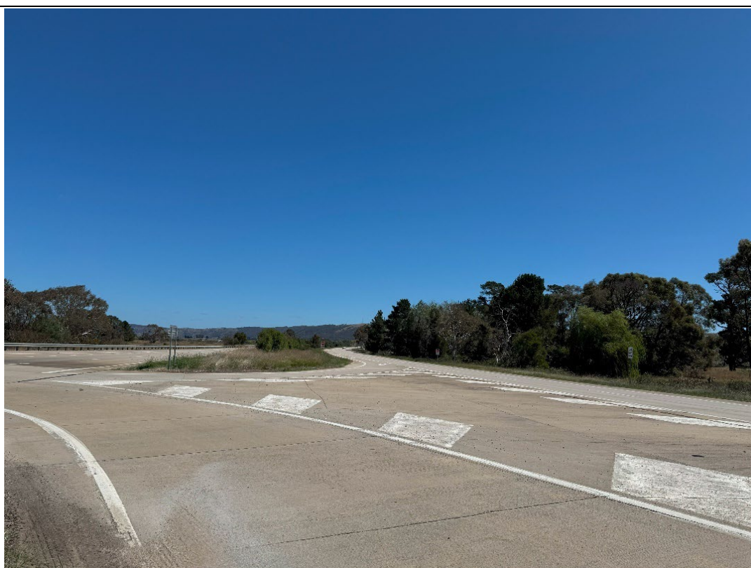
Figure 6 Site Access Federal Highway looking North
