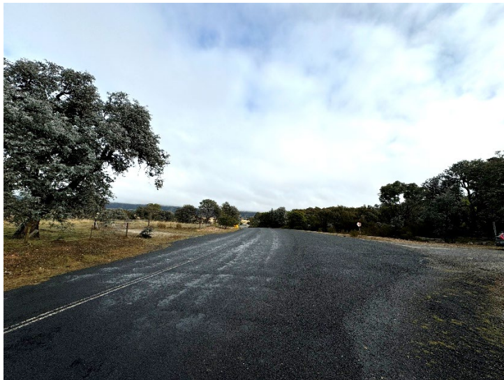
Photo 4-2 Collector Road – View from East of Site Access to West
