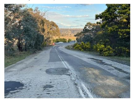
Existing surface of Collector Road – 9 September 2025 – road is clearly not wide enough for trucks and surface is poor.
