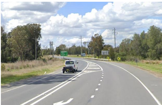
Figure 2-10 Elizabeth Drive, facing east (Source: Google Earth)
