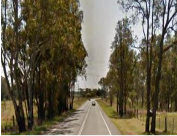
Figure 2-4 Luddenham Road, facing north
