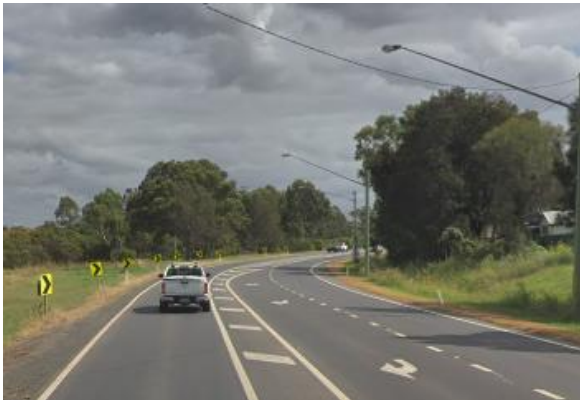
Figure 2-8 Mamre Road, facing north (Source: Google Earth)
