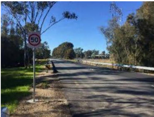
Figure 2-6 Patons Lane, facing west
