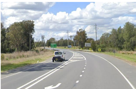
Figure 2-9 Elizabeth Drive, facing east (Source: Google Earth)
