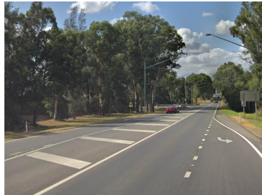
Figure 2-8 Mamre Road, facing south (Source: Google Earth)
