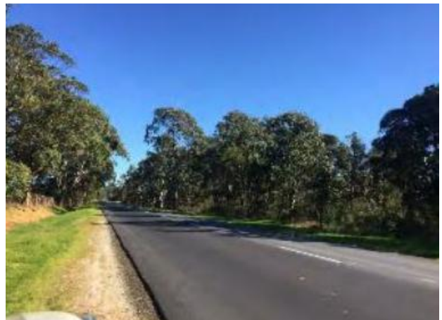
Figure 2-6 Patons Lane, facing east
