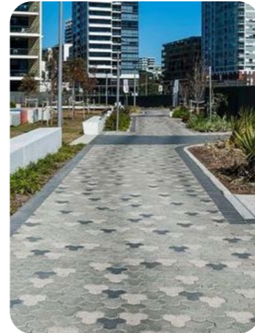
P5: Trafficable Stone Pavers
