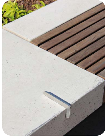
SW - Concrete seating wall
