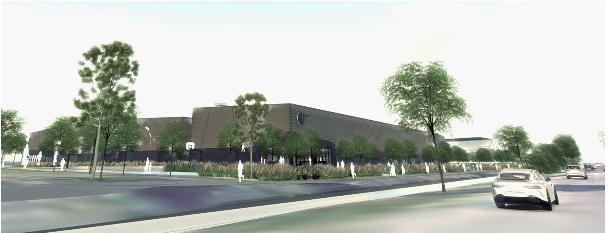
Figure 84 - Original SSDA Image – West-South-Western View from Monash Rd West (Aug. 2024)
