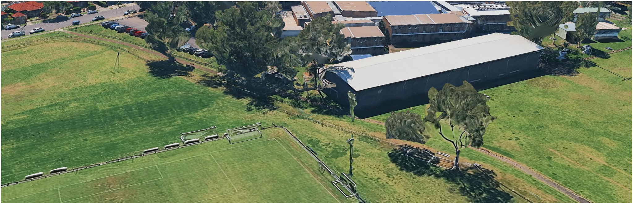
Figure 93 – Existing Pedestrian Access from NW of Subject Site to Wombain Rd (source: Google Maps 3D)
