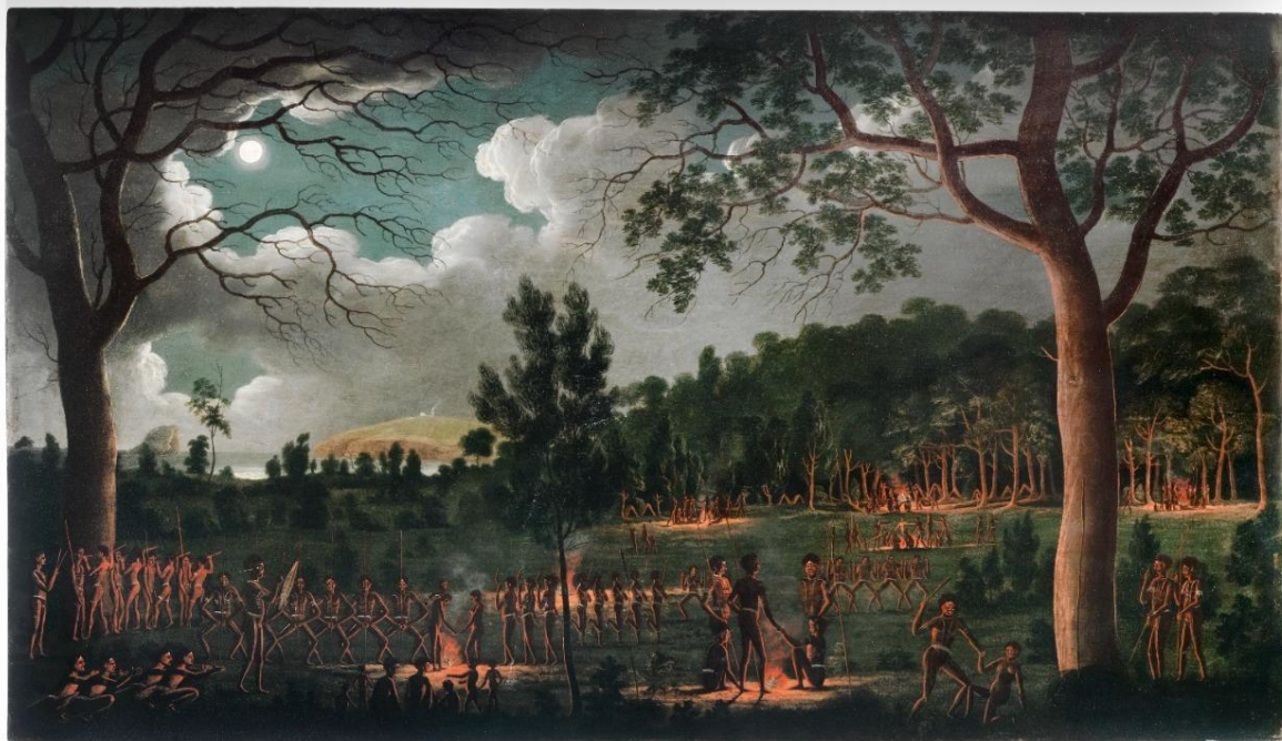
Figure 5. Corroboree at Newcastle, 1818 (Source: State Library of NSW)
