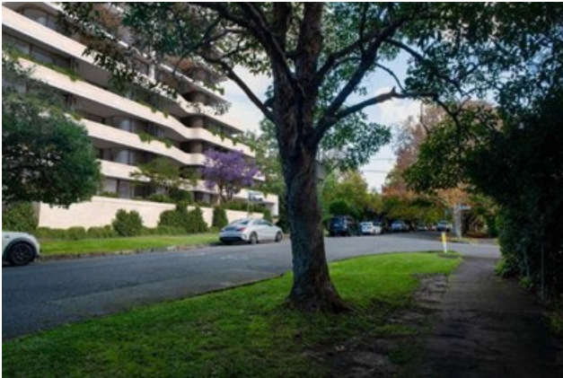
Figure 29 McIntosh Street view looking west.
