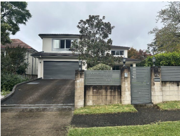
Picture 13 25 McIntosh Street, showing the high fence and modern features.
