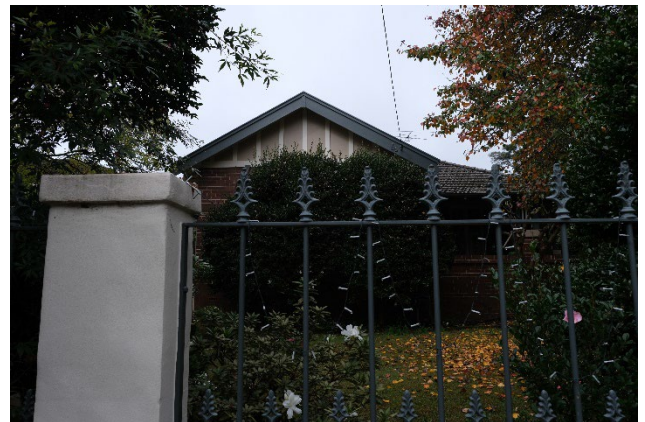
Picture 10 Fence and infilled street facing gable end.
