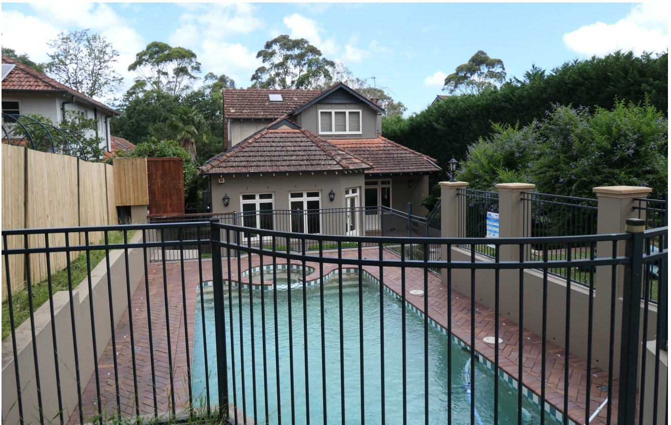
Figure 15 The rear of 19 Balfour Street
