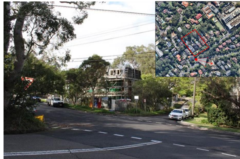
Figure 12: Looking south west from the side of 23 Bent Street (Source: Keylan)
