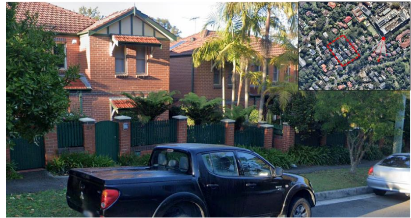
Figure 8: Facing south towards 24 Balfour Street (Source: Google Maps)
