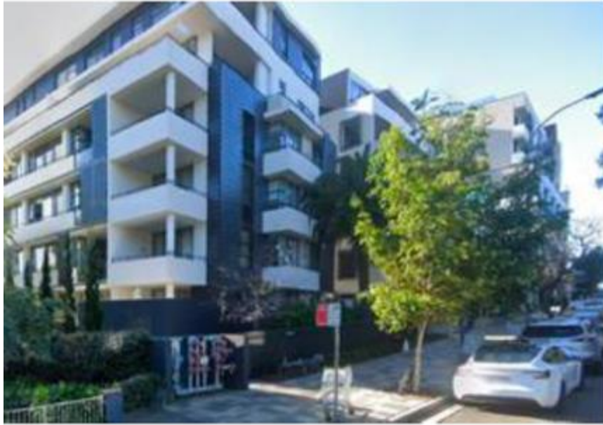
5-6 storey residential flat building in Lindfield Avenue
