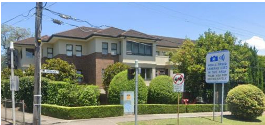
Residential flat building corner of Grosvenor Road & Pacific Highway Lindfield
