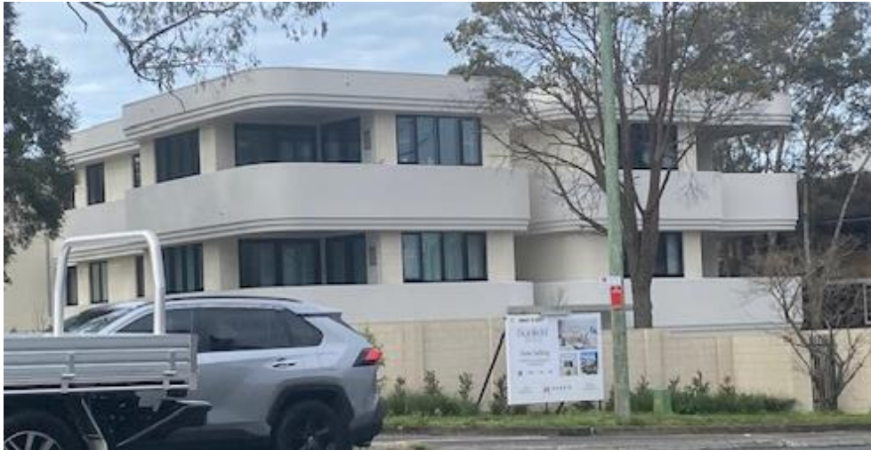
Recently constructed RFB cnr Eton Road & Pacific Highway Lindfield
