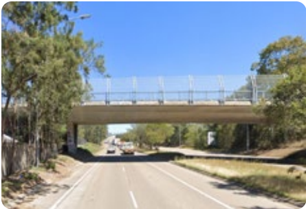
Above: Janet St overpass of Newcastle Inner City Bypass - 5.25m height clearance
