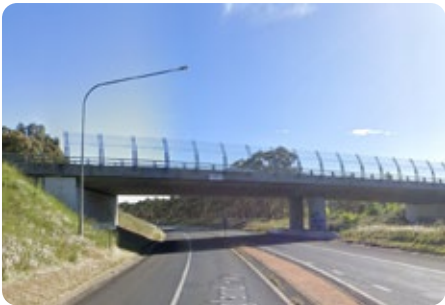
Below: Queen Elizabeth Dr overpass of New England Hwy at Armidale - 4.9m height clearance
