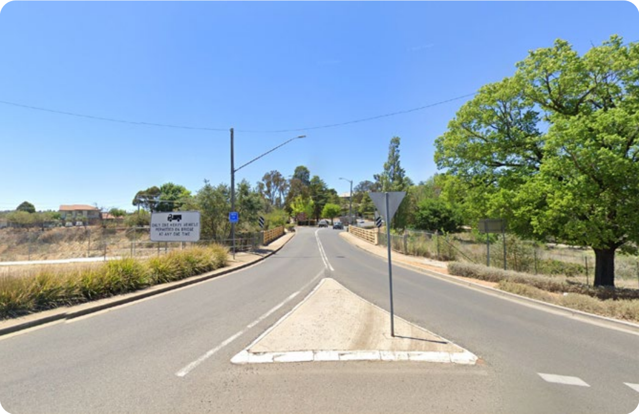
Above: Kentucky St rail overpass in Armidale
