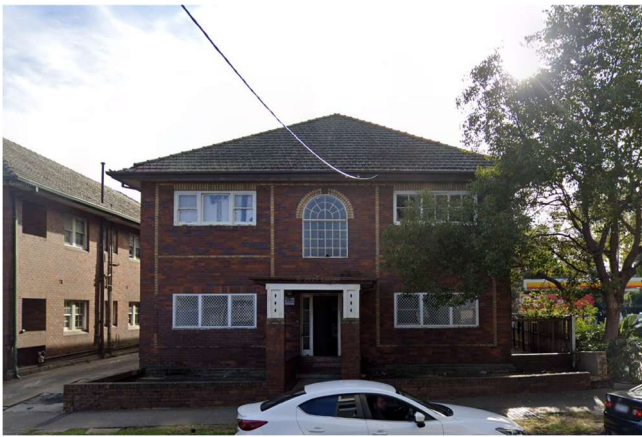
Figure 28 External photograph of 11 Albert Road.
