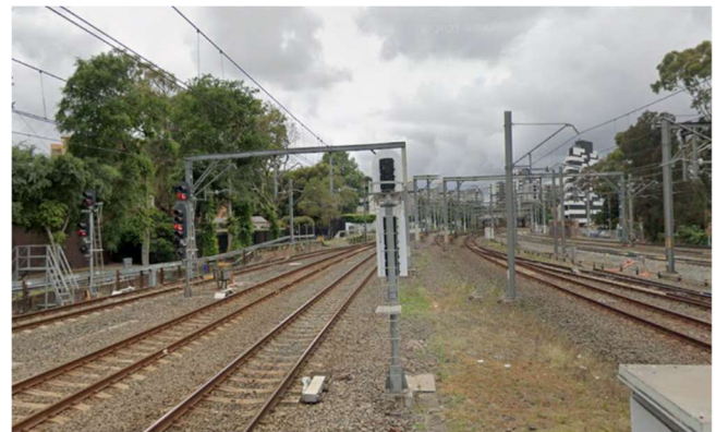
Figure 9 External photograph from Strathfield platform towards the subject site
