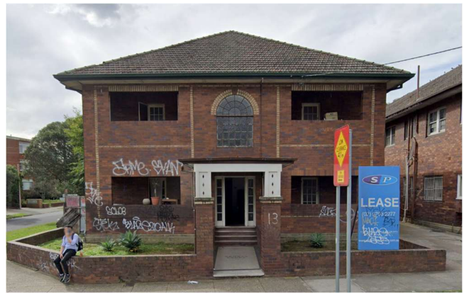
Figure 29 External photograph of 13 Albert Road.
