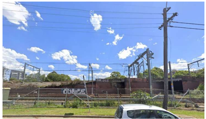
Figure 7 External photograph of Cooper Street and Strathfield railway line showing part of heritage listed railway flyovers.
