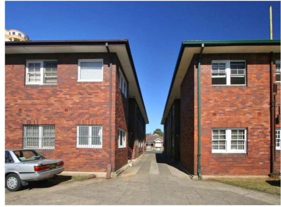
Figure 27 External (rear) photograph of 11 (left) & 13 Albert Road (right).
