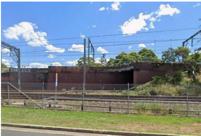
Figure 35 External view of the Strathfield Flyover
