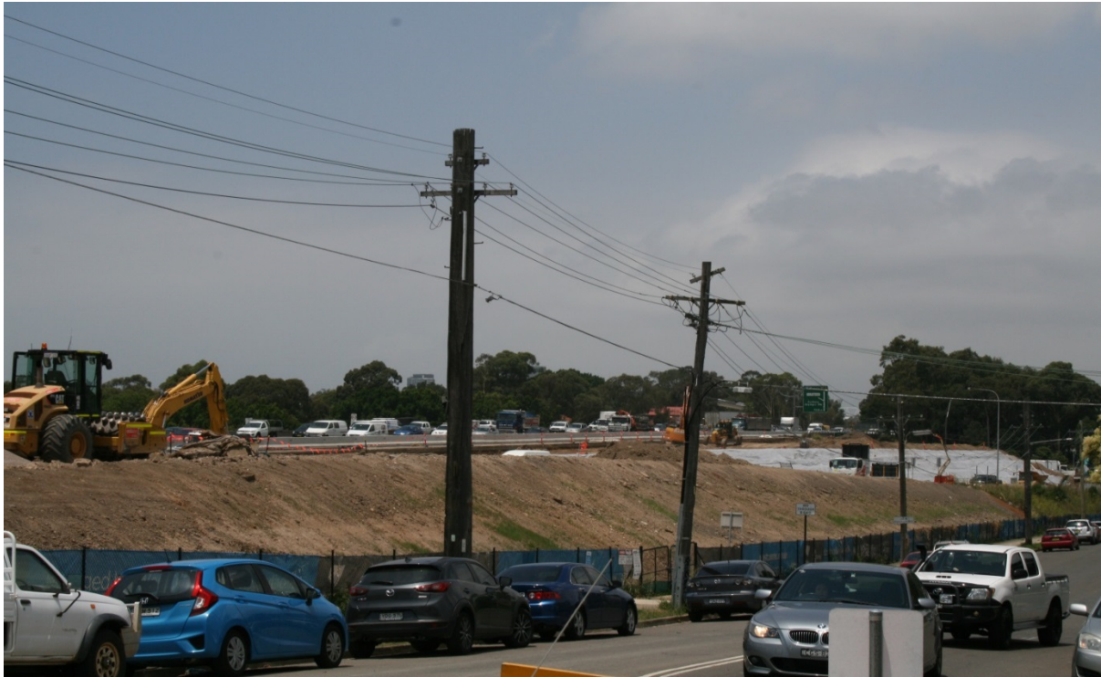
(Photo by V. Elton 10/12/2015 – construction zone Adderley St, Auburn)
