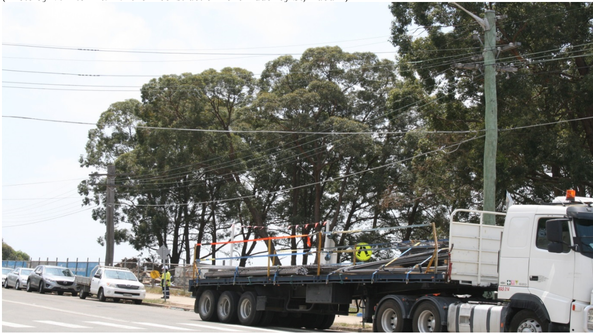
(Photo by V. Elton 10/12/2015 Adderley St towards M4 construction zone. The Ibis nesting tree is towards the rear of the truck)
