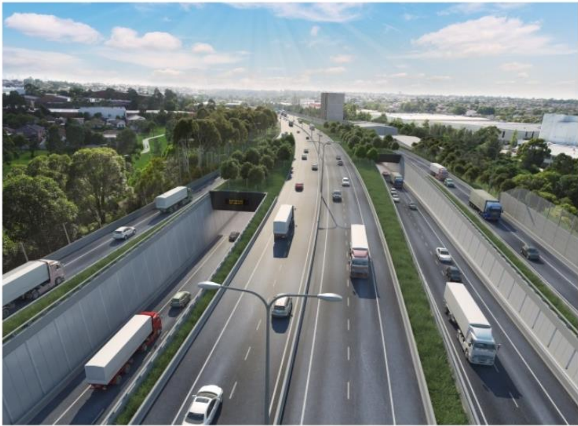
Figure 3 – M5 East entry and exit portals looking east
