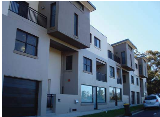
Fig 9. Live/work precedent at Lilyfield Rd, Lilyfield fronting railway line
