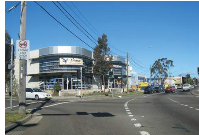
Fig 31. Contemporary built form addressing street corner
