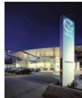
Fig 30. Prominent and well-defined signage on street frontage
