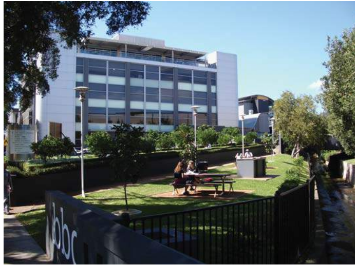
Fig 1. Open space fronting canal for worker amenity
