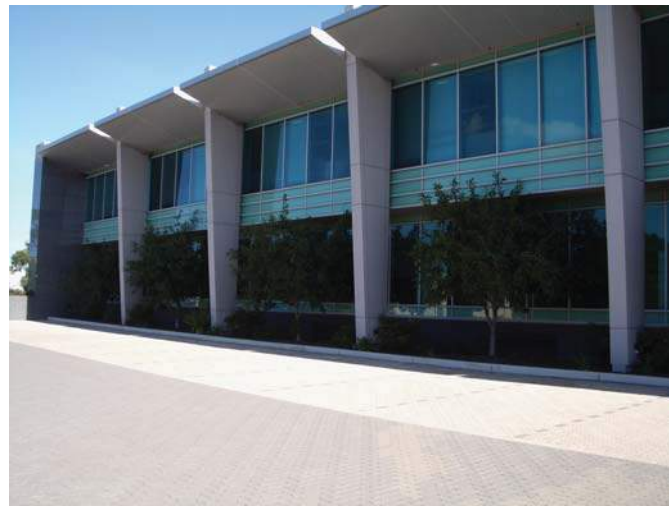
Fig 15. Eaves overhang, fins articulate facade
