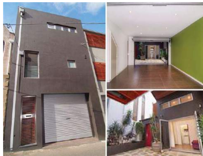
Fig 12. Studio on ground level with garage roller doors and living on upper levels - Redfern
