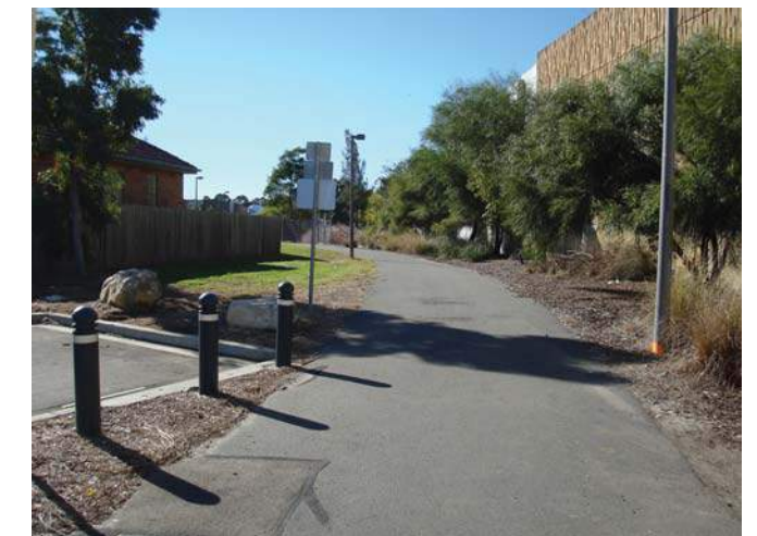
Fig 36. Well-landscaped pedestrian link along M5
