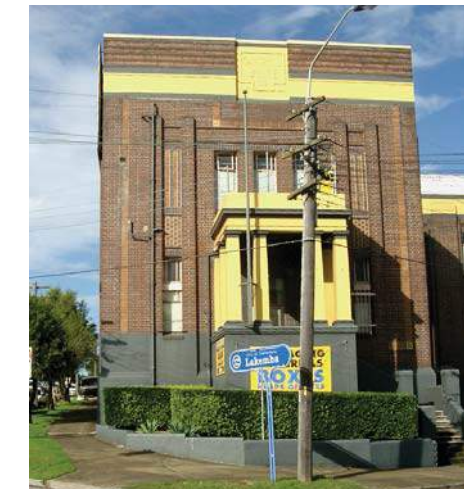
Fig 34. High quality existing industrial building should be retained
