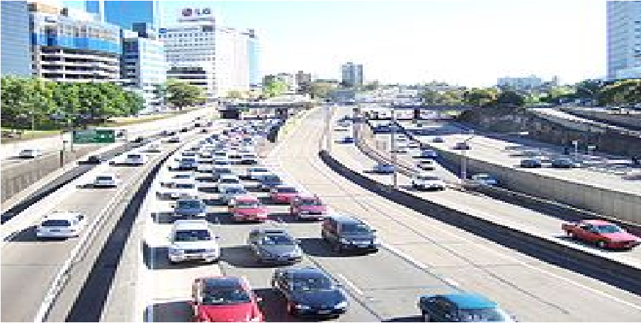
Warringah Freeway looking north, over the inner western carriageway.
