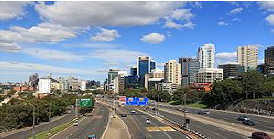
Warringah Freeway looking south at its widest point - 16 lanes
